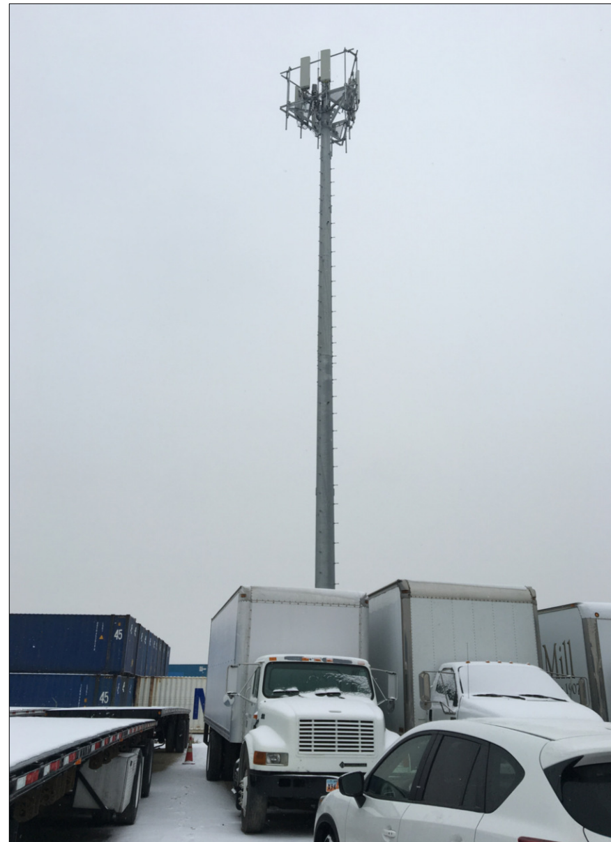
VIEW OF EXISTING TOWER (LOOKING EAST)
