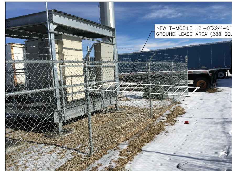
VIEW OF NEW EQUIPMENT AREA (LOOKING NORTHEAST)
